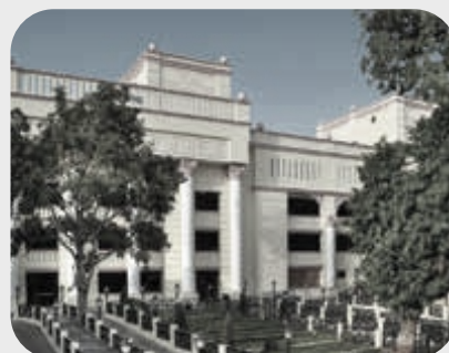
MULTILEVEL PARKING HAZRATGANJ
