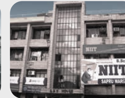
SAS HOUSE SAPRU MARG
